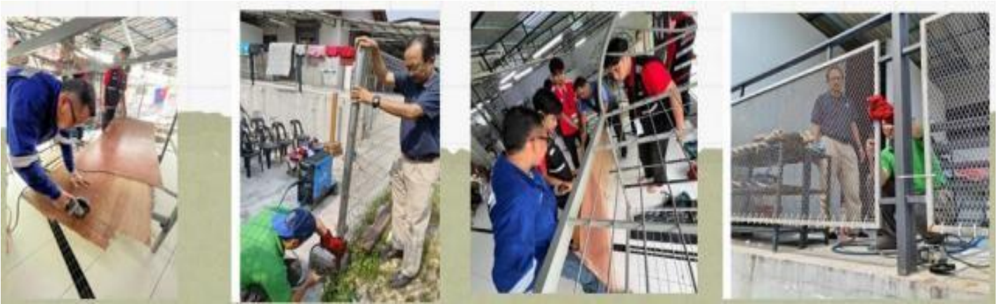
Figure 3: shows the repair activities of Fitra Qaseh facilities by JKM PIS.
